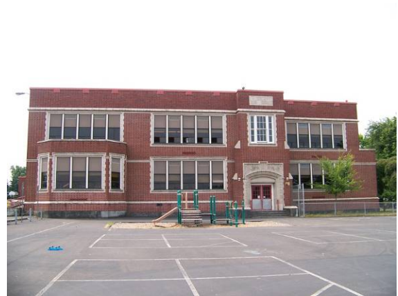
Main building (294A), north (side) elevation, looking south.
