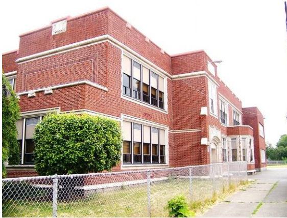
Main building (294A), west (front) and south (side) elevations, looking east.
