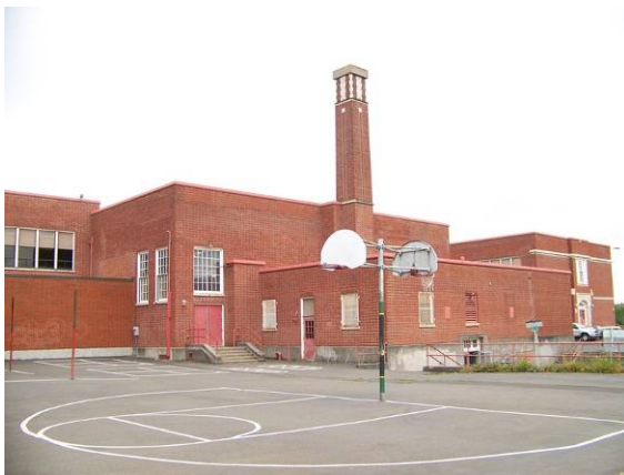
Main building (294A), east (rear) elevation, looking northwest.
